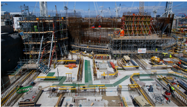
Fig 8. Hinkley Point C Nuclear Power Plant. Image Source: Bloomberg
