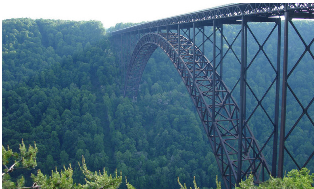
Fig 5. West Virginia’s New River Gorge Bridge. Image Source: Burgess & Niple.
